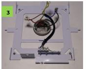
Connect the Smart-Connect base wiring to the light circuit.
