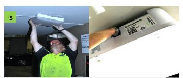
Place Smart-Connect Base plate hinge tabs into slots located at opposite end to barrel lock. Align the electrical connector terminal pins on the light fitting to the terminal block sockets on the base.
