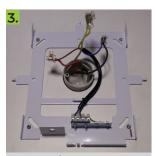
Connect the Smart-Connect base wiring to the light circuit. Emergency lights must be connected to permanent active and must not be switched, to prevent premature battery failure.
