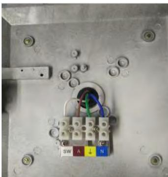
5. Connect building wiring to mains terminal.
