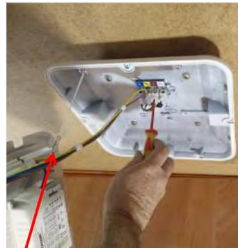
6. Use hook provided to suspend gear tray from base and connect gear tray wiring (see next images).
