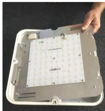
9. Hook gear tray under metal bar and swivel locks to secure the gear tray.
