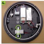
Unscrew the battery mounting bracket, and replace old battery with new and connect to the driver
