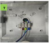
Connect wire loom from gear tray into the terminal block.
