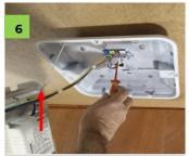
Use hook provided to suspend gear tray from base and connect gear tray wiring (see next image).
