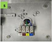
Connect building wiring to mains terminal.
