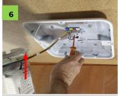
Use hook provided to suspend gear tray from base and connect gear tray wiring (see next images).
