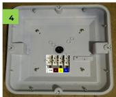
Mount base to the surface. If IP65 rating is required use cable gland & side entry on the side opposite the LED driver and seal screw holes.
