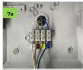
Connect Switched Active into **SW** terminal, Permanent Active into **A** terminal. See note on bottom of page.
