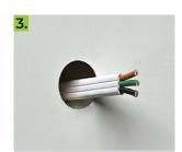
Remove the bracket to show the hole markings. Drill mounting holes and a 20mm hole for the cable entry
