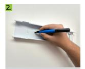
Place the mounting bracket at the ceiling/wall location, allowing 50mm on each side for its sliding mechanism. Mark the position of the screw holes and cable entry through the bracket
