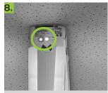
After installation, this fitting is now a fully operational emergency light, please check indicators on the side of the fitting.
