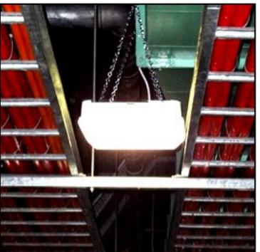
Once installed, the Chameleon can be easily detached from the Smart-Connect base without disconnecting the power, making it easy for maintenance or light replacement.
