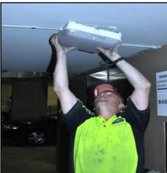
4. Place Smart-Connect Base plate hinge tabs into slots located at opposite end to barrel lock. Once aligned, press the light upwards to connect. Push barrel lock in to secure.
