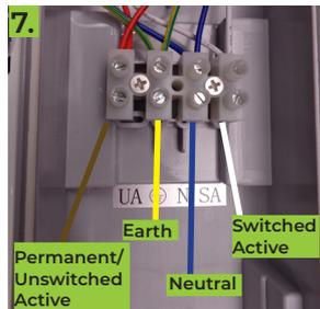
Wiring of emergency fitting with switched and unswitched active present
