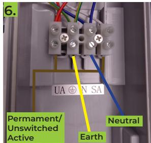
Wiring of emergency fitting with only unswitched active present. Insert loop between UA and SA terminal.
