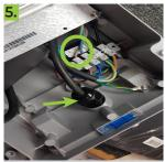
Connect mains wires to terminal block. Tighten cable gland.
