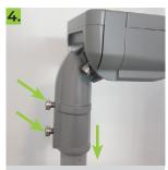
Feed cable into light fitting, slip pole adaptor over pole and secure by tightening the bolts to 17 Nm. Do not overtighten.
