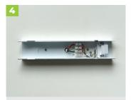
Feed the cables through the holes of the mounting bracket and connect the cables into the terminal block.
