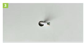
Remove the bracket to show the hole markings. Drill a 20mm hole for the cable entry. Install the bracket. Make sure the mounting screw locations are against solid material to support the weight of the fitting.
