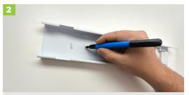
Place the mounting bracket at the ceiling/wall location. Mark the position of the screw holes and cable entry through the bracket.
