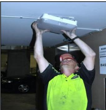
4. Place Smart-Connect Base plate hinge tabs into slots located at opposite end to barrel lock. Align the electrical connector terminal pins on the light fitting to the terminal block sockets on the base.
