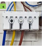
Connect Neutral wire to terminal "N", Earth to earth terminal, active wire to terminal
