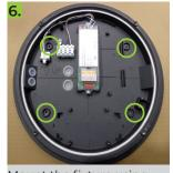
Mount the fixture using the 4 mounting holes indicated. For wall mounting, ensure the fitting is mounted with the ↑ pointing up
