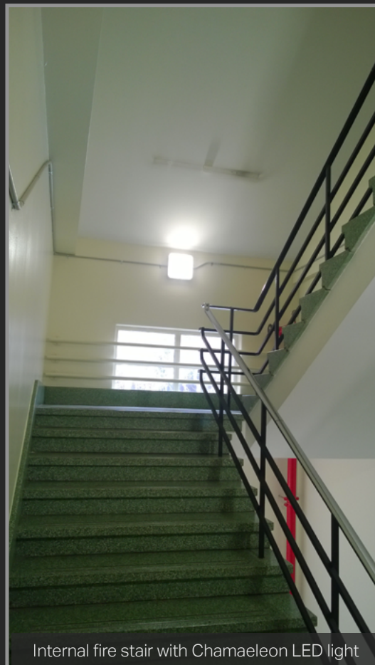
Replacement of Twin T8 Fluorescent tube & 10W non maintained emergency batten with a single Chamaeleon light
