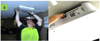
Place Smart-Connect Base plate hinge tabs into slots located at opposite end to barrel lock.
