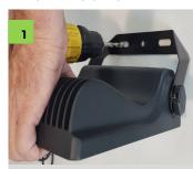
Drill mounting holes. M10 fixing size is recommended
