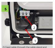
(1) Feed cable through the cable gland and tighten cable gland (2) Connect wires to terminal block. Max cable size 2.5mm². Outer sheath diameter up to
