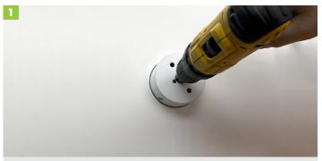
Mark the position of the fitting at the desired ceiling location and provide a 75mm - 150mm diameter cutout
