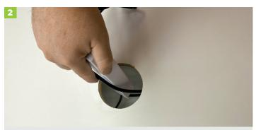
Pass the inverter and battery pack through the cutout and secure it against a solid structure e.g. beam or truss using screws. Guide the supplied flex cable through the cutout and connect the plug to mains power
